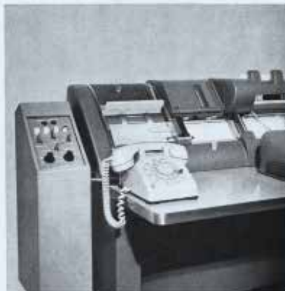
At the data processing center, an IBM Card Punch receives data by phone and automatically punches it into a card, ready for processing.
